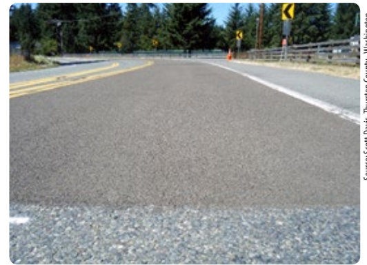
HFST at Thurston County Horizontal Curve Demonstration Site
